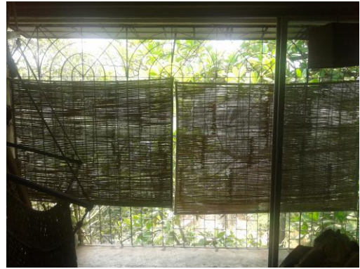
Figure 4: After installation and rolling down of chicks to reduce window area.
